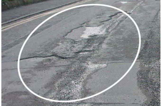
Damage type = potholing
