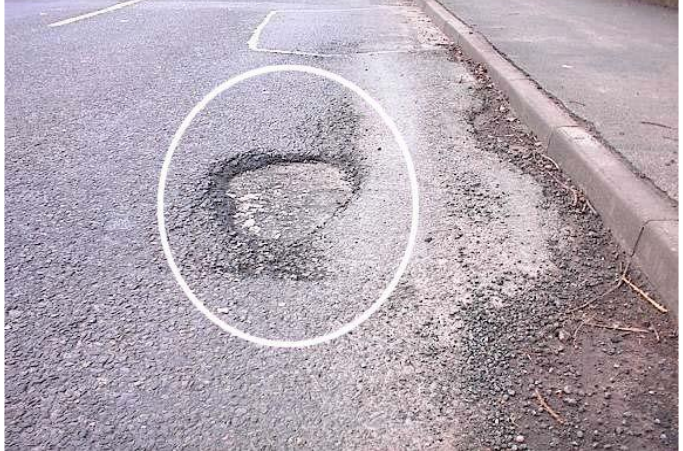
Damage type = potholing
