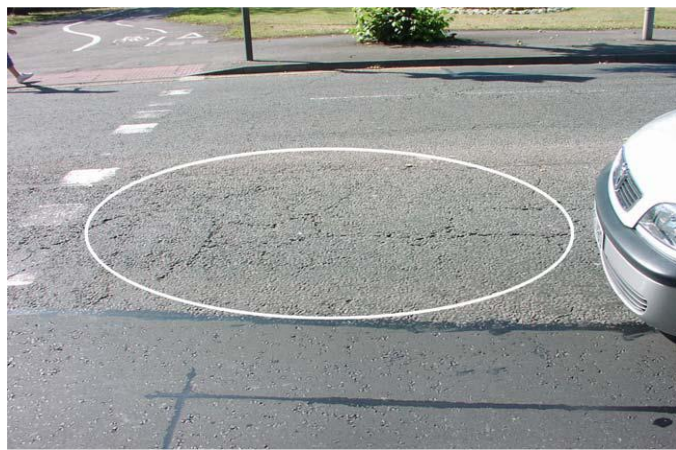
Damage Type = subsidence
